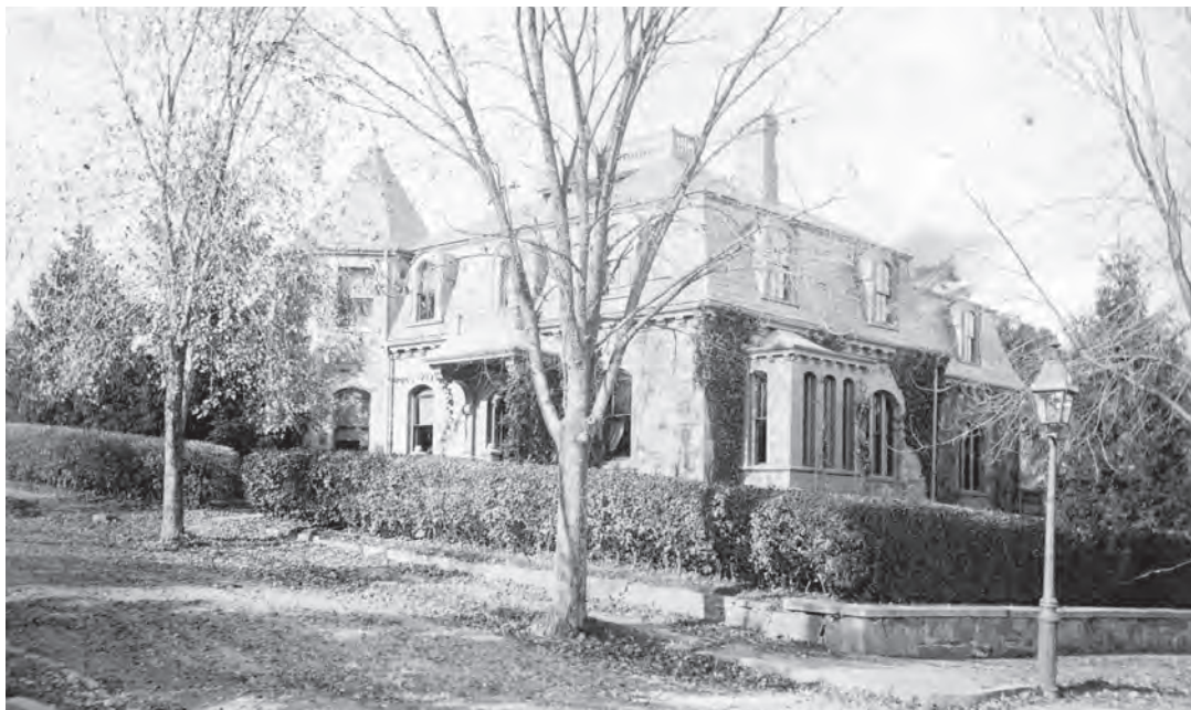
Chase home at Alton Place and St. Paul Street
